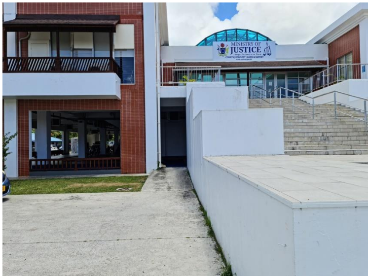
Frontal view of the lift location with the opening to the east of the stairway
