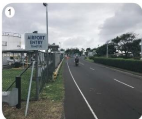
Poor pedestrian access to airport
